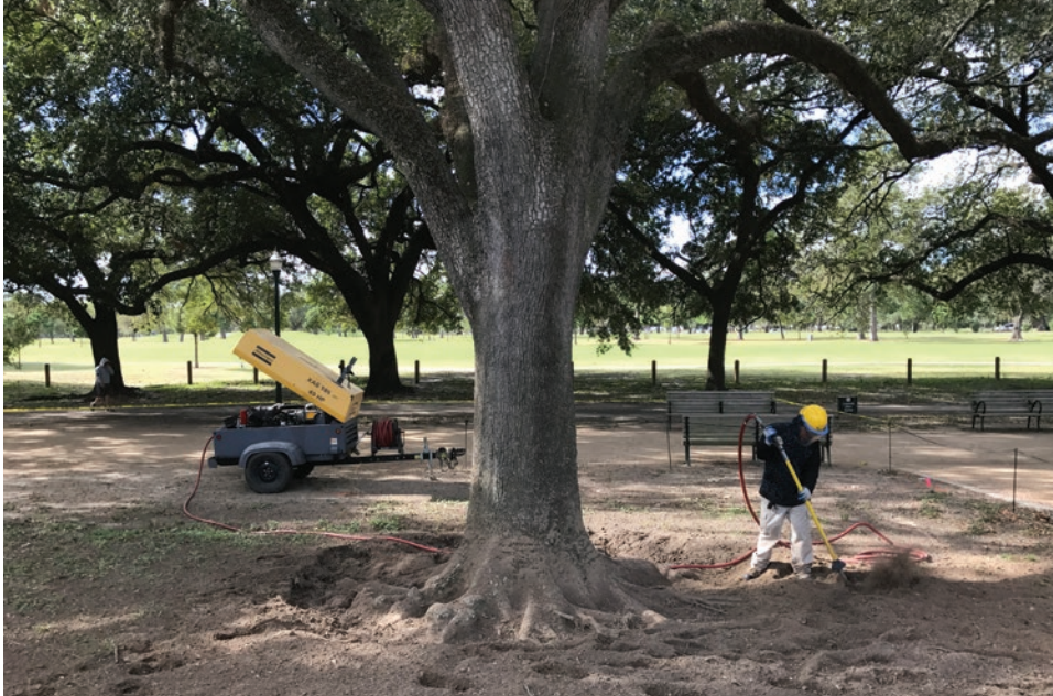
Bartlett Tree Experts air spading the soil surrounding the affected trees
